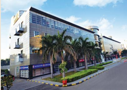
FIRST INDIA PLACE MG Road, Gurugram Operational Area 1,72,908 sq ft
