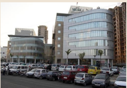
VATIKA ATRIUM Golf Course Road, Gurugram Operational Area 2,36,000 sq ft
