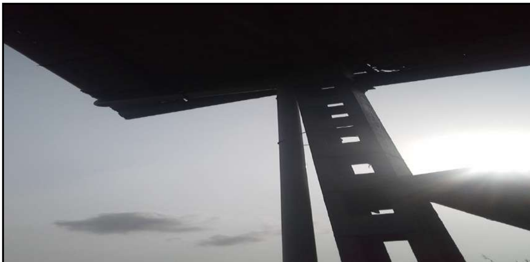
Figure 5.2 Rain Water Harvesting on site of TDMCCL
