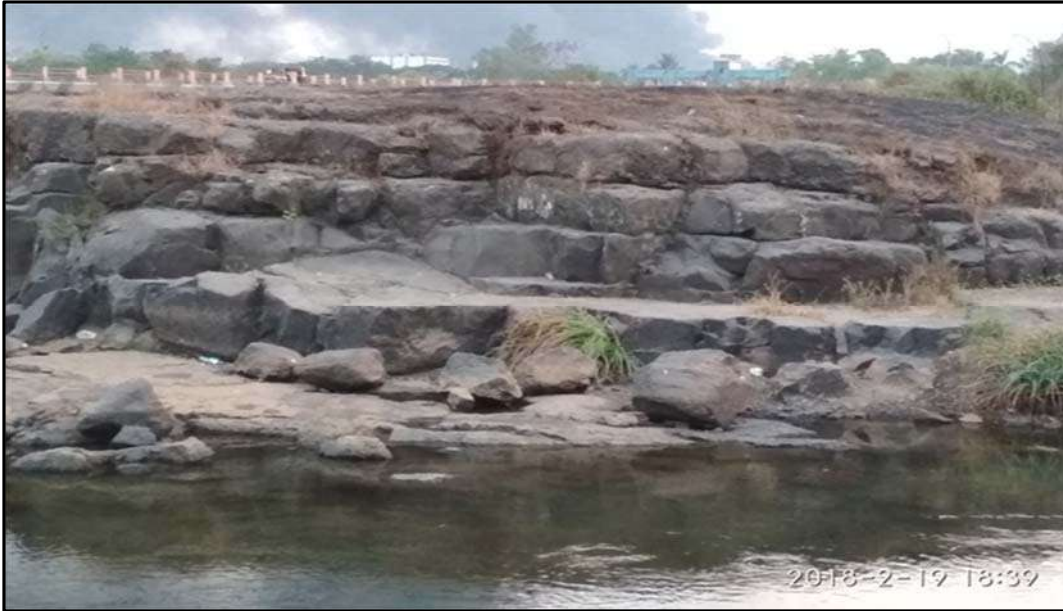
Plate 2 Compact basalt with sheet joints in left bank of Kundalika River, Dhatav
