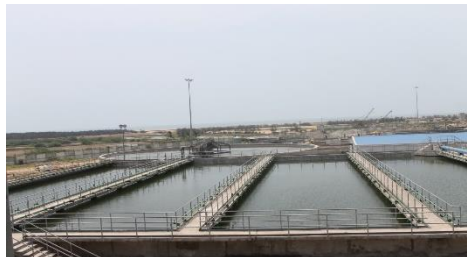
54 MLD Effluent Treatment and recycling plant, for Indian Oil Corporation Limited, Paradip, Odisha, India India's largest industrial water recycling plant
