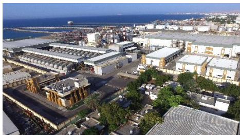
191 MLD SWRO (Desalination) Plant, Al Gubrah, Oman Largest desalination plant in the country of Oman
