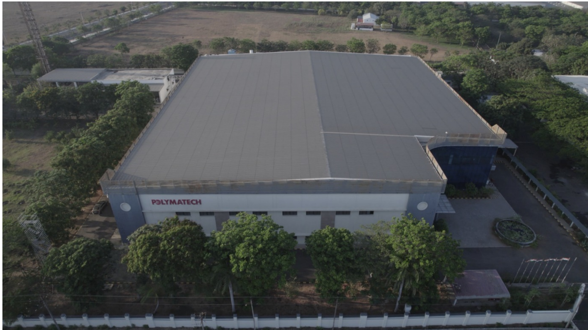
Our manufacturing plant at Oragadam, Kancheepuram, Tamil Nadu.
