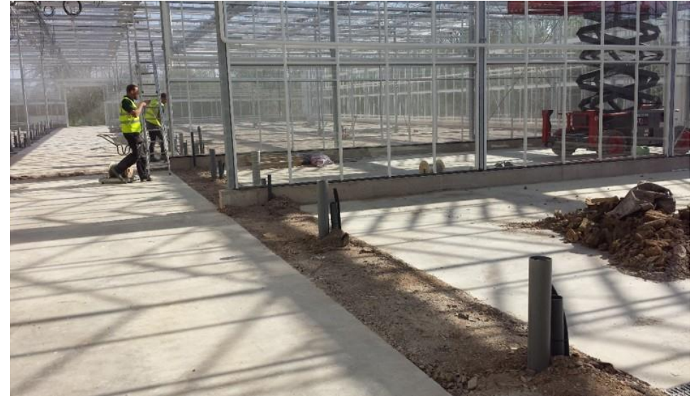
Ebb and flood irrigation pipework
