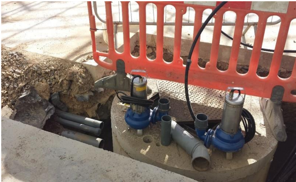
Flood and ebb sump tanks
