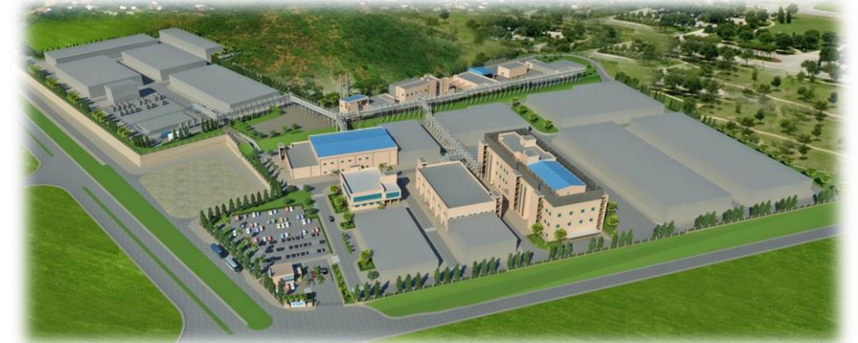
Syngene's API manufacturing facility at Mangaluru
