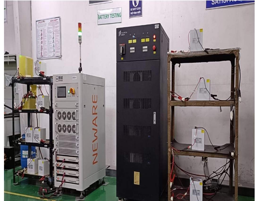
Battery Capacity Testing Machine
