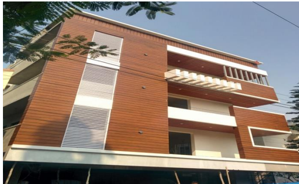
Cement Planks Cladding Apartment Complex – Bangalore
