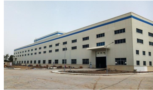
Taikai Electric India Ltd. – Savli, Gujarat
