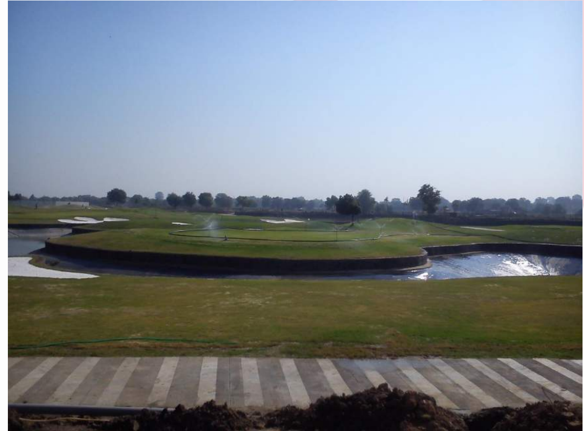
Golf Course Construction
