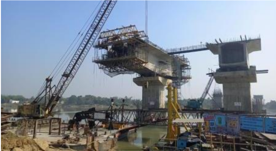
Bhagirathi bridge super structure works at Baharampore Bypass
