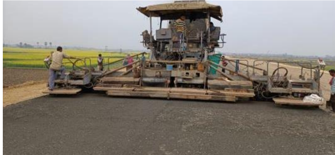
Road works at Baharampore Bypass
