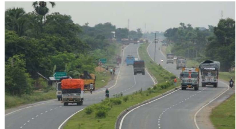
Km 341 (Farakka Raiganj Highway)
