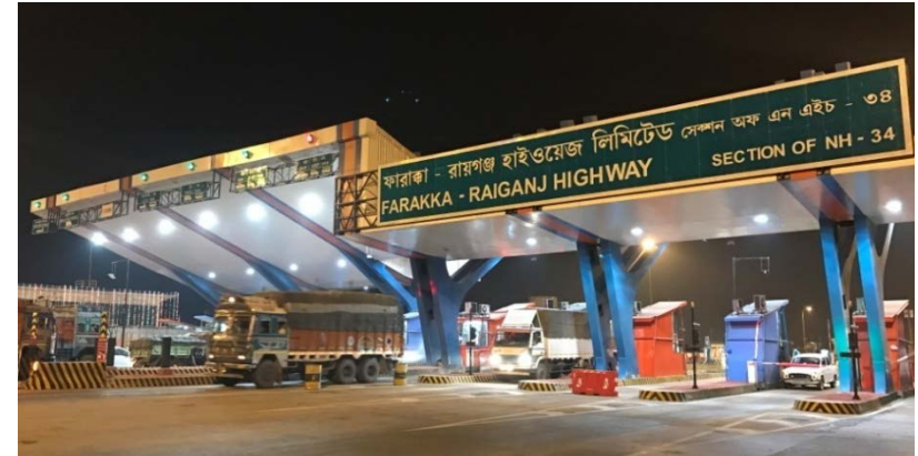
Farakka Raiganj Highway: Toll Plaza at Km 297
