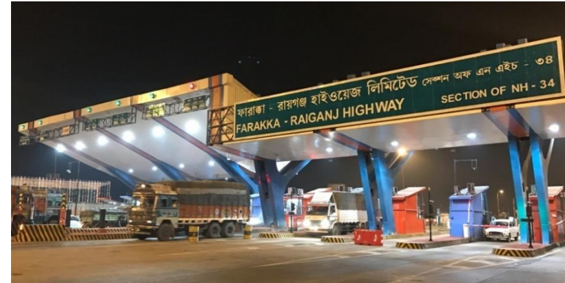
Farakka Raiganj Highway: Toll Plaza at Km 297
