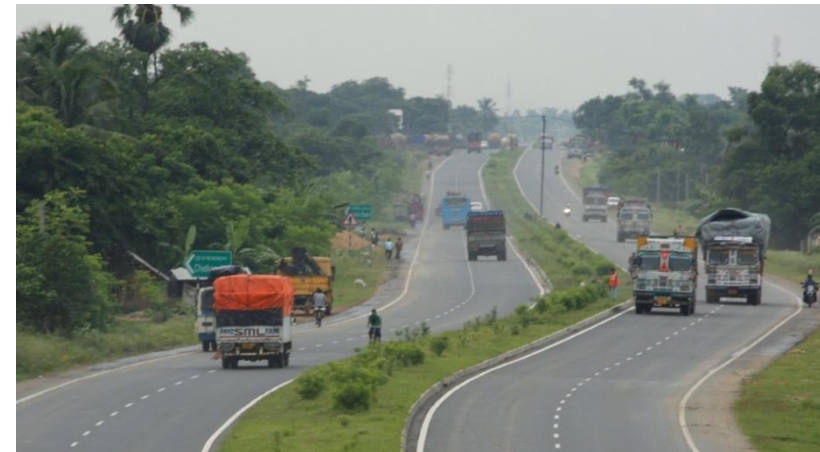
Km 341 (Farakka Raiganj Highway)
